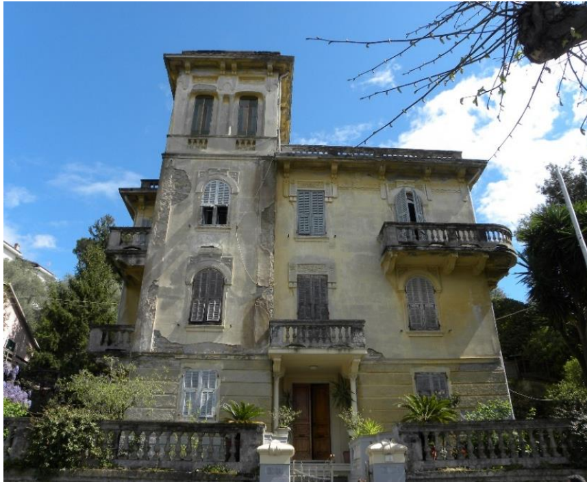
Figure 3.1.– Building's frontal view.
