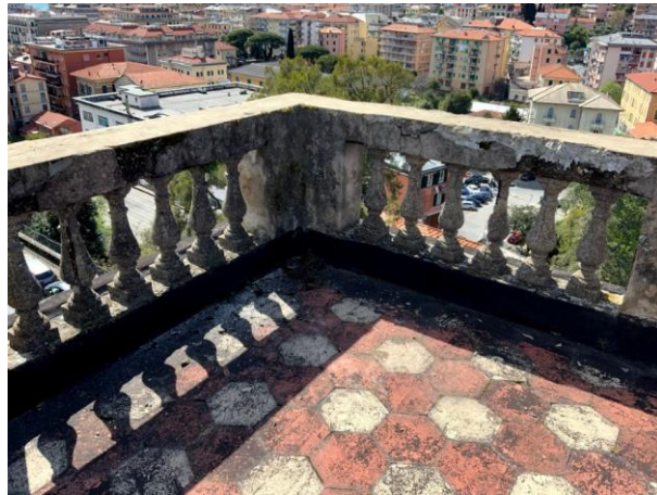
Figure 3.10- Particular parapet on the roof
