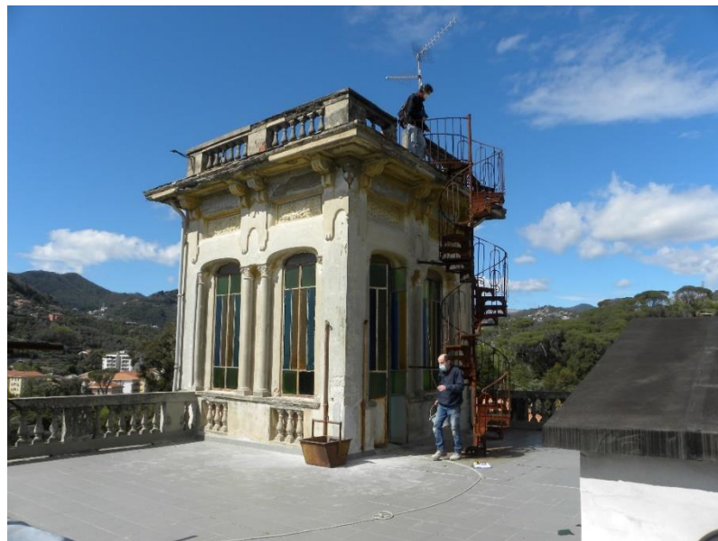
Figure 3.9 – Flat Roof and tower
