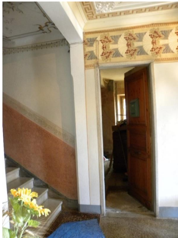
Figure 3.5 - Ground floor interior, beam detail.
