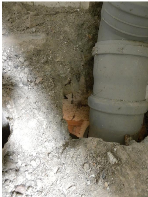
Figure 3.15 - Investigation on the interfloor slab.
