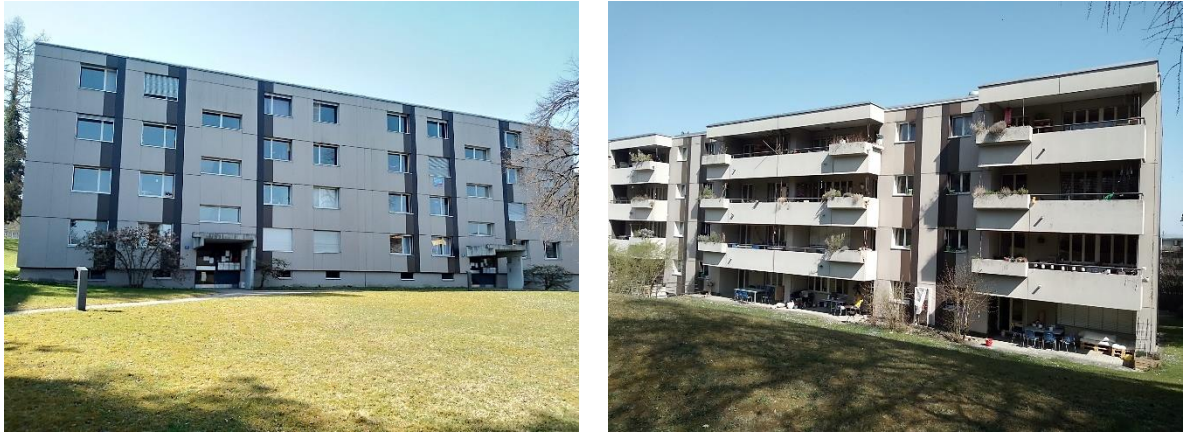
Figure 2: Eastern façade (left), western façade with balconies (right)
