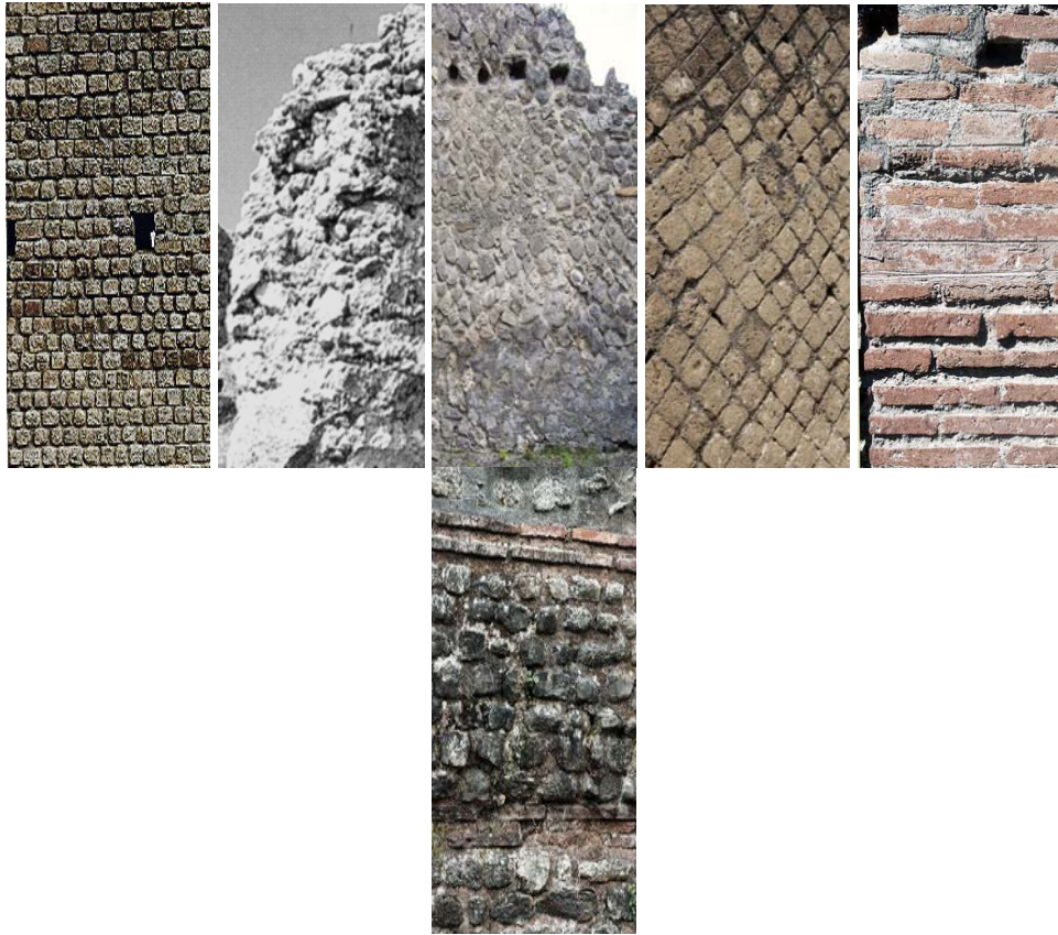
Fig 1.8 opus quadratum; opus caementicium; opus incertum; opus reticulatum; opus latericium; opus mixtum
