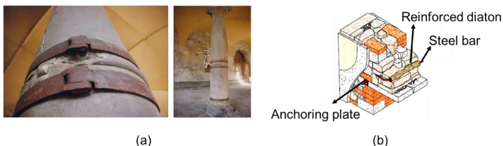
Figure 4.23. Discrete confinement of a: (a) pier and (b) multi-layer wall (adapted from EU-India cross program, 2006).
