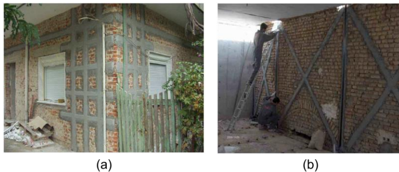
Figure 4.22. FRP application examples: (a) grid pattern (Sika Limited, 2003) and (b) shear strengthening on one side (Motavalli, 2005).
